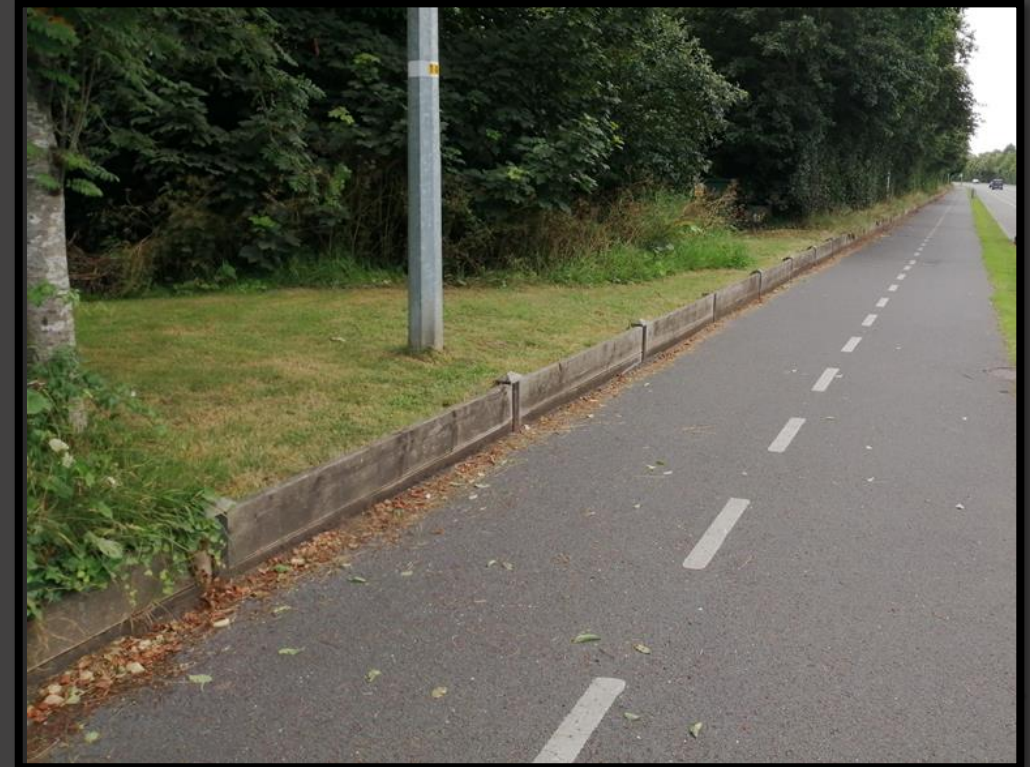
Ring Road footpath & cycle lane
