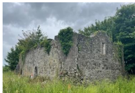
Dunkitt church walls will be stabilised
