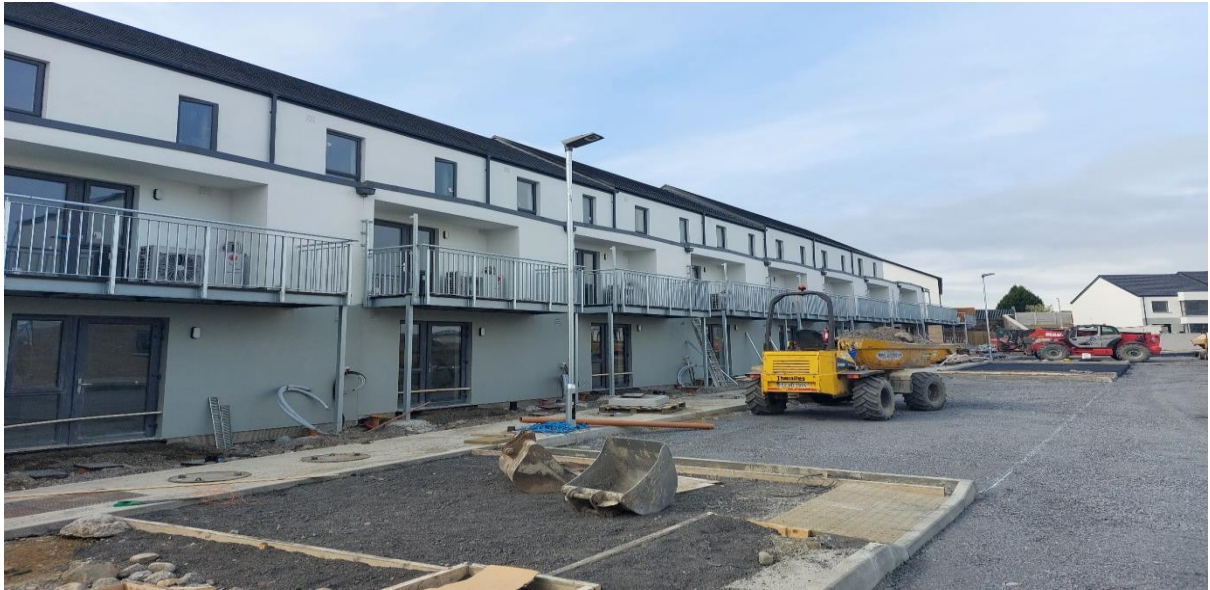
Works on Pennefeather Green nearing completion
