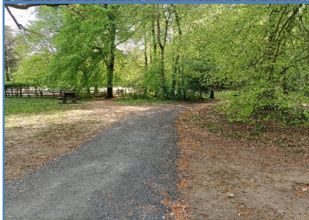
Improvements to footpaths underway in Woodstock
