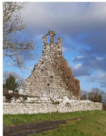
The bell tower at Clomantagh Church will be repaired
