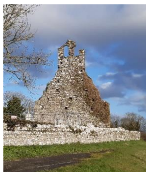
The Bell Tower at Clomantagh Church will be repaired
