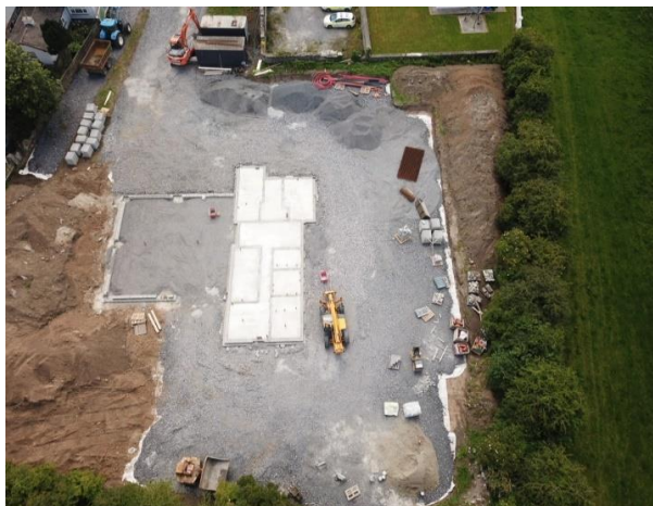
Aerial photo shows the foundation for the new Fire Station.
