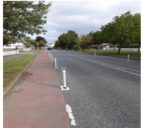
Provision of Cycle Bollards on Bohernatounish Road
