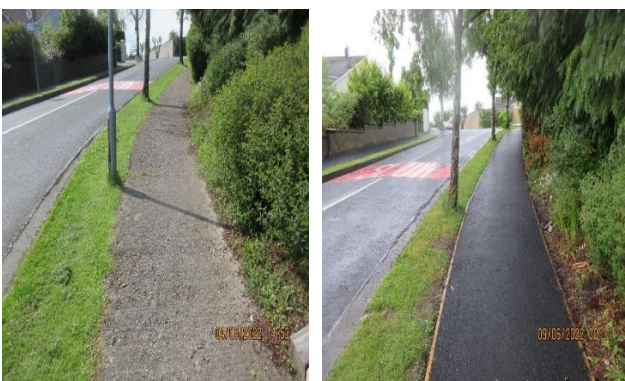
Footpath Repairs At Glendine Before & After
