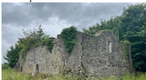
Dunkitt Church walls will be stabilised
