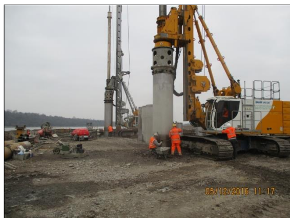
Piling Works at Pier 3 at Pink Rock.
