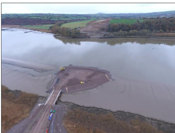
Barrow Bridge - Temporary Impermeable Working Area for Pier 4
