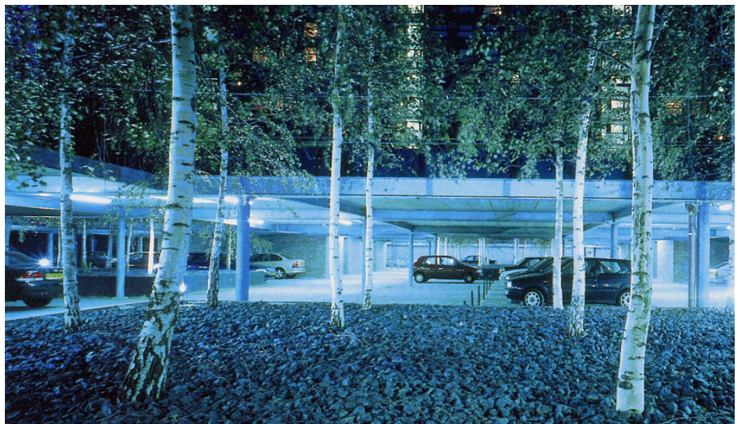
Covered car parking
