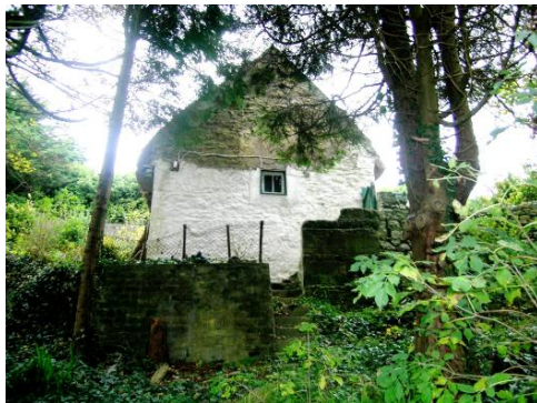
Side of cottage
