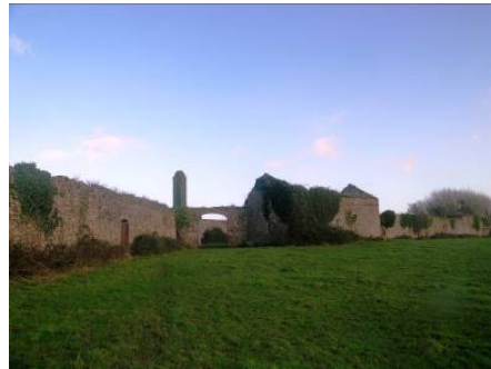
View of outbuildings
