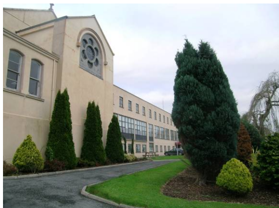
Church & new development alongside
