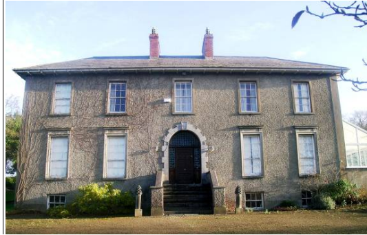
Main entrance façade
