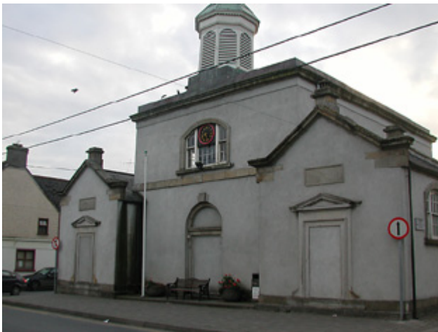
Fig 6.2: Castlecomer Court House
