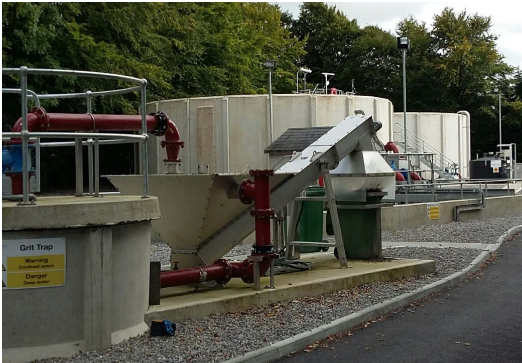
Figure 8.1 Wastewater Treatment Plant Upgrade
