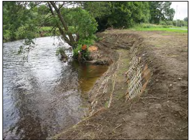
Plate 4.1 – Riverbank restoration along the Nore (Photo: G. Smith)
